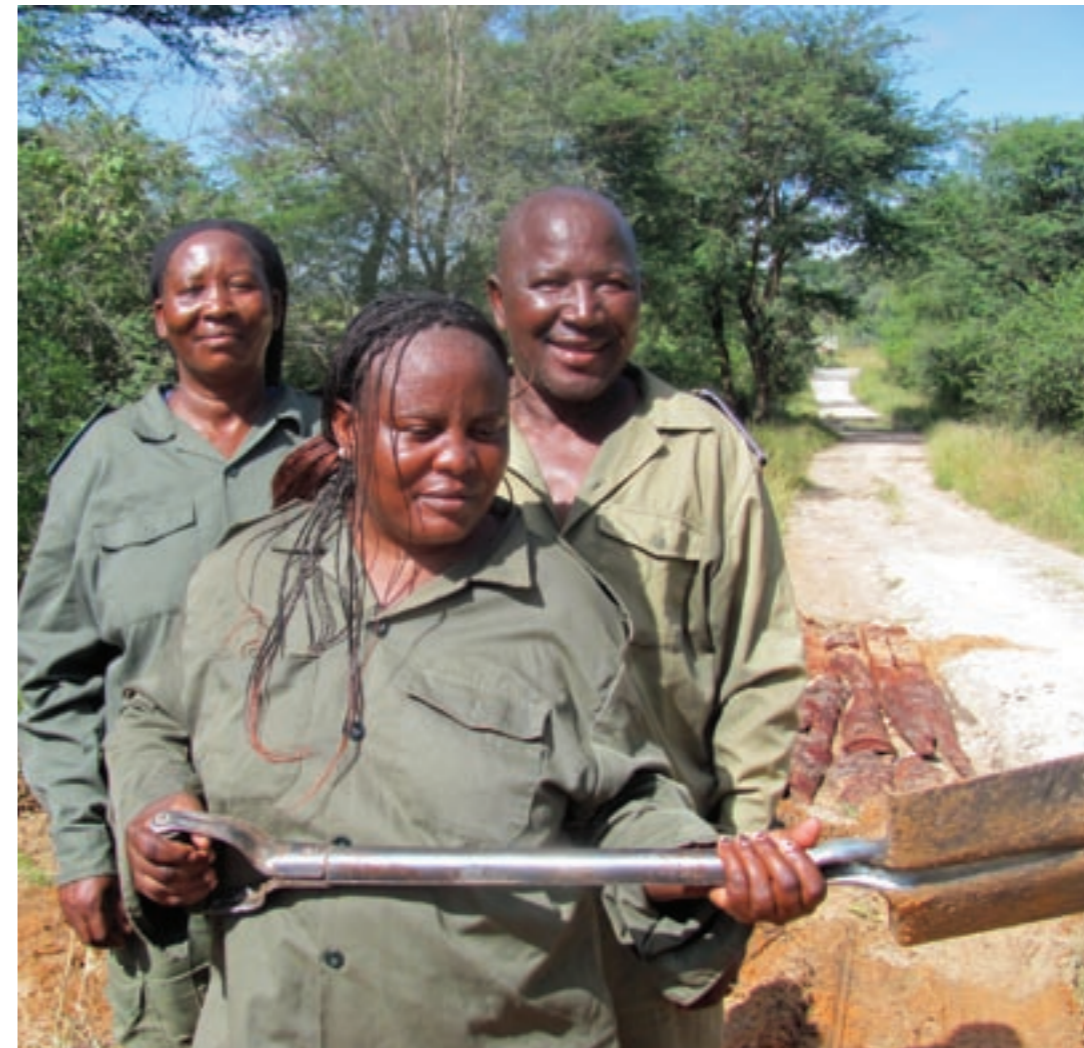
MET staff are the custodians of Namibia's PAs on behalf of the citizens of the country. Here Bwabwata National Park staff are repairing the tourist road to Susuwe Station.
