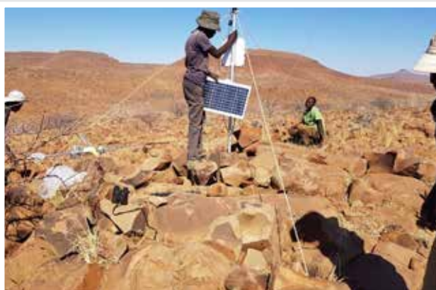
Figure 33: An early-warning logger being installed by MEFT staff, October 2021.
