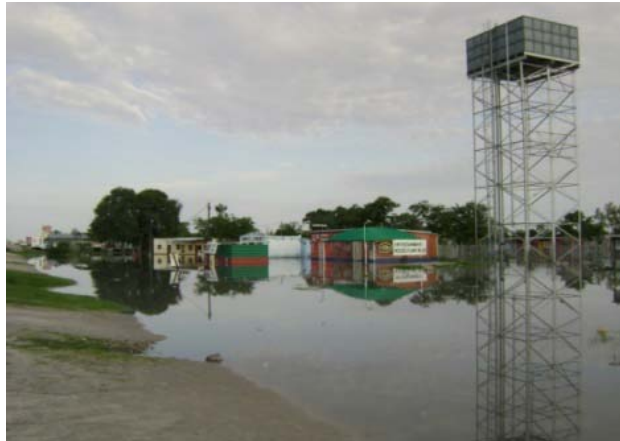
Figure 19: Flooding in a local village, Omusati
