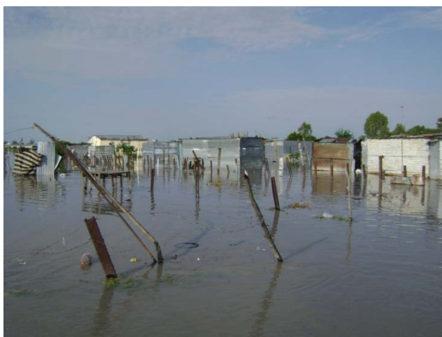
Figure 25: Flooding of houses built of corrugated iron
