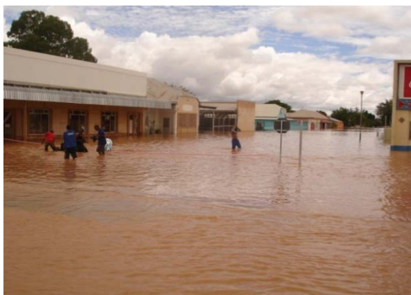
Figure 5: Houses affected by flooding
