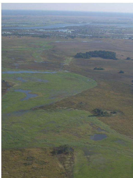
Figure 30: Arial view of flooding
