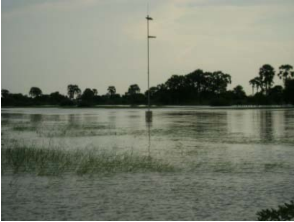
Figure 8: Flooding occurred in three of the past five years
